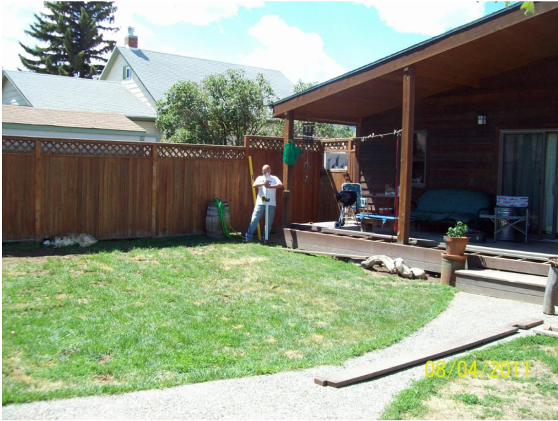
View northeast of porch, backyard and east end of house 512 Adams Avenue South, Red Lodge, MT 100_2686.JPG
