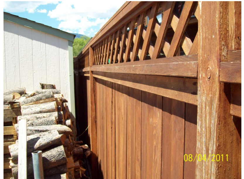
View west of fence between properties and green house 518 Adams Avenue South, Red Lodge, MT 100_2689.JPG
