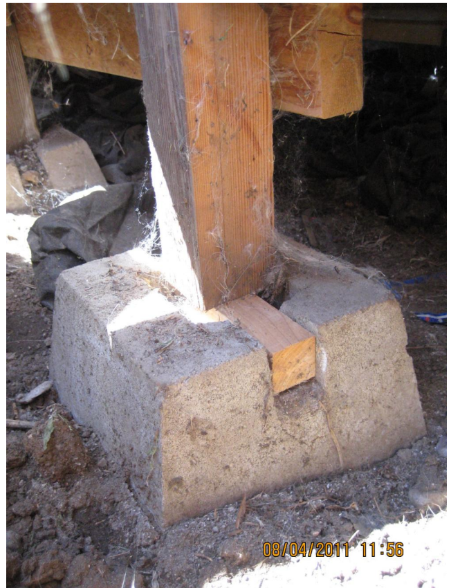
View of concrete block and wood shim below the back deck along east side of house. Photo by DEQ-AML 512 Adams Avenue South, Red Lodge, MT 512 Adams St._8-4-11 005.jpg
