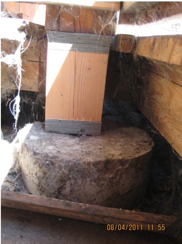
View of concrete pier and wood shim below the back deck along east side of house. Photo by DEQ-AML 512 Adams Avenue South, Red Lodge, MT 512 Adams St._8-4-11 004.jpg
