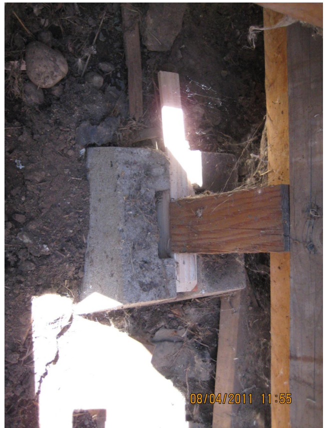
View of concrete block and wood shim below the back deck along east side of house. Photo by DEQ-AML 512 Adams Avenue South, Red Lodge, MT 512 Adams St._8-4-11 002.jpg
