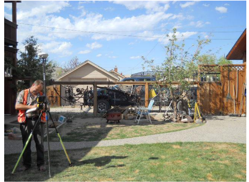
8/22/2011 4:01:00 PM View north of backyard; surveyor standing near area of settlement 512 Adams Avenue South, Red Lodge, MT 2011-0062.JPG
