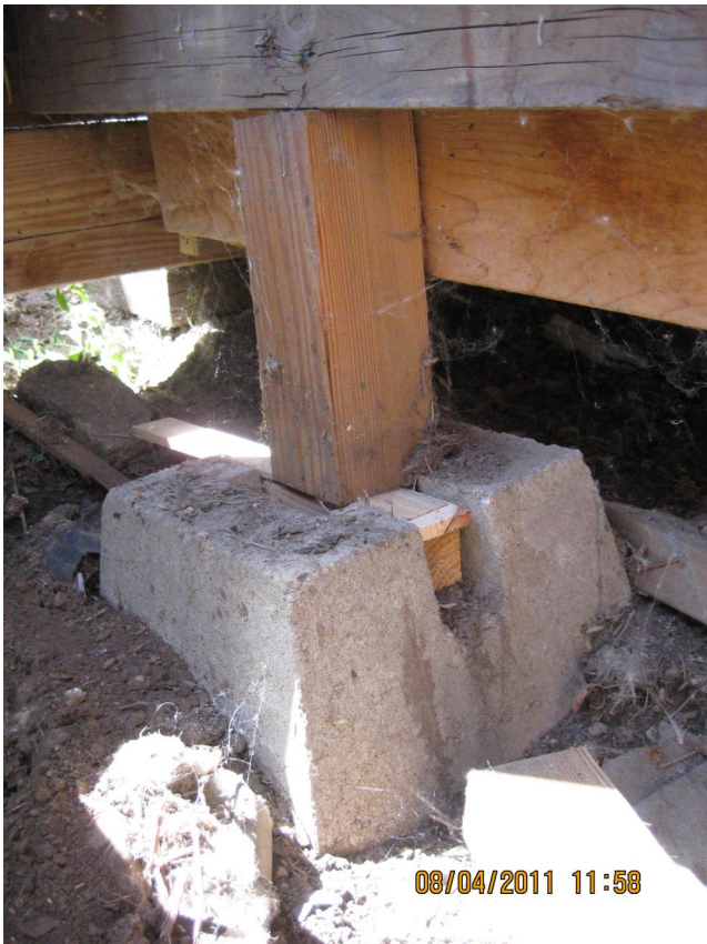
View of concrete block and wood shim below the back deck along east side of house. Photo by DEQ-AML 512 Adams Avenue South, Red Lodge, MT 512 Adams St._8-4-11 006.jpg
